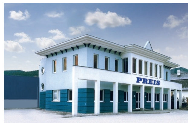
The Headquarter in Pernitz / Austria
